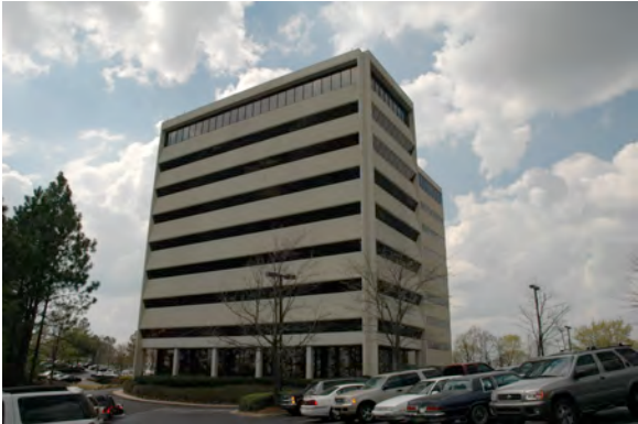
Beacon Ridge Tower
